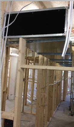
Exhaust duct installation
