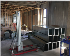
Commercial air duct installation
